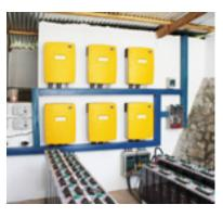
This section Climate and Resource Protection for Economic Development project seeks to provide a smart energy efficiency and management solution for buildings. The system is designed to manage power supply from different sources (PV, Grid and bio-fuel generator) to meet the load requirements of the buildings (LT and Professorial blocks) to maximize reliability of supply. The system consists of smart meters, sensors, relays and switches which are controlled by an intelligent
